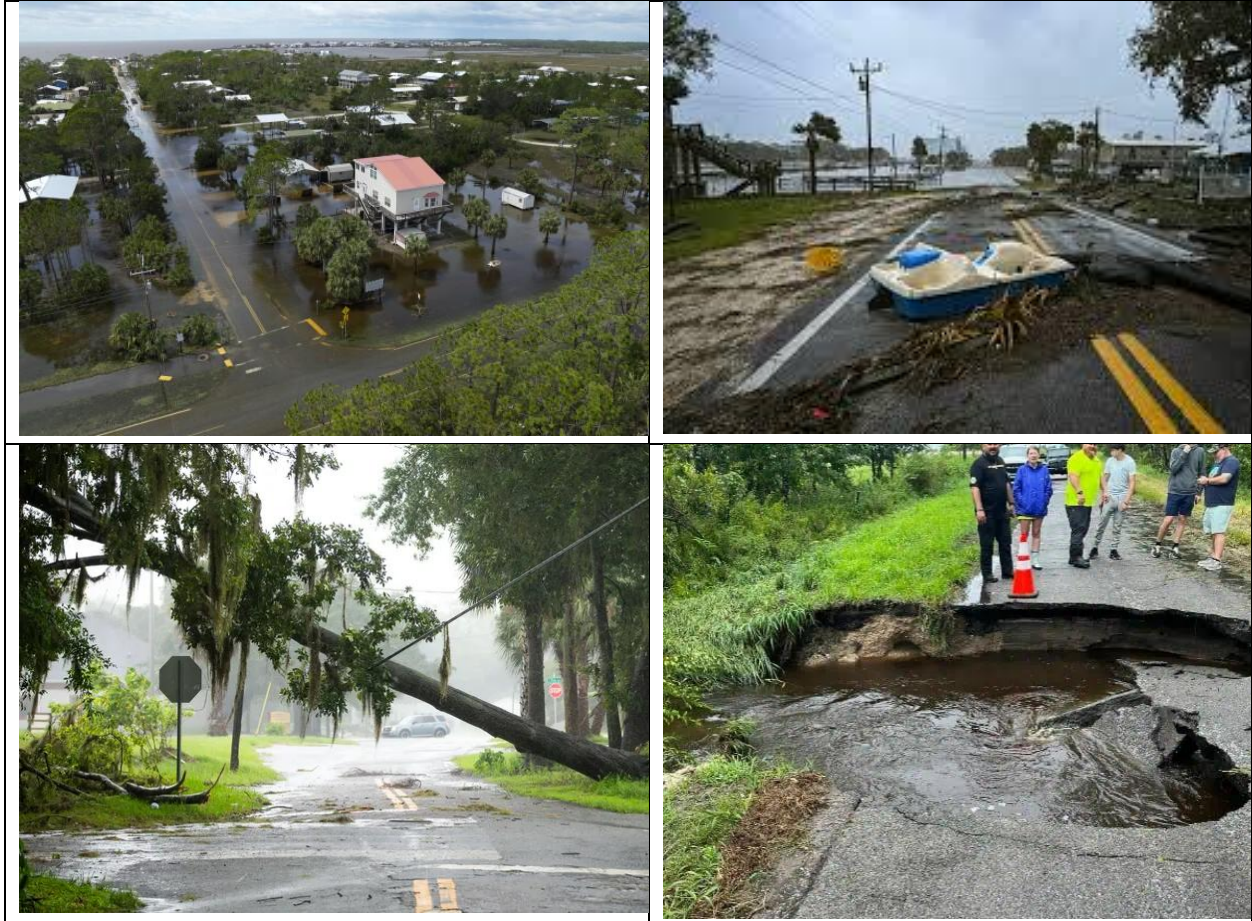
Figure 3:2 Images of Damage Caused by Hurricanes Idalia and Debby on Roadway Infrastructure ( “https://www.tampapf.com/hurricane-debby-leaves-severe-damage-in-florida-sen-rubio-and-rep-cammack-urge-full-federal-assistance/#google_vignette” 2024)
