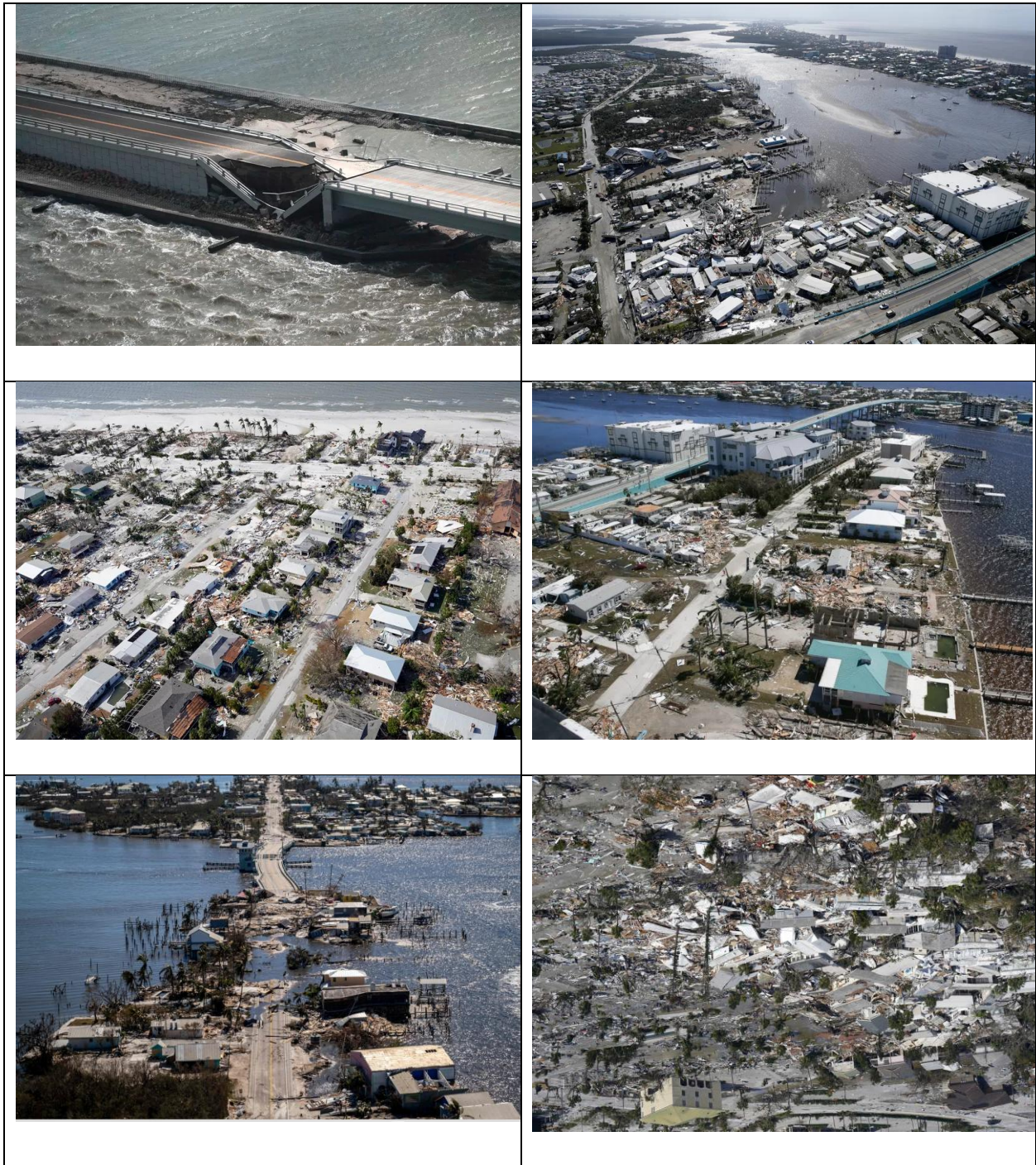
Figure 2:2 Images of Damages Caused by Hurricane Ian on Roadway Infrastructure (27)
